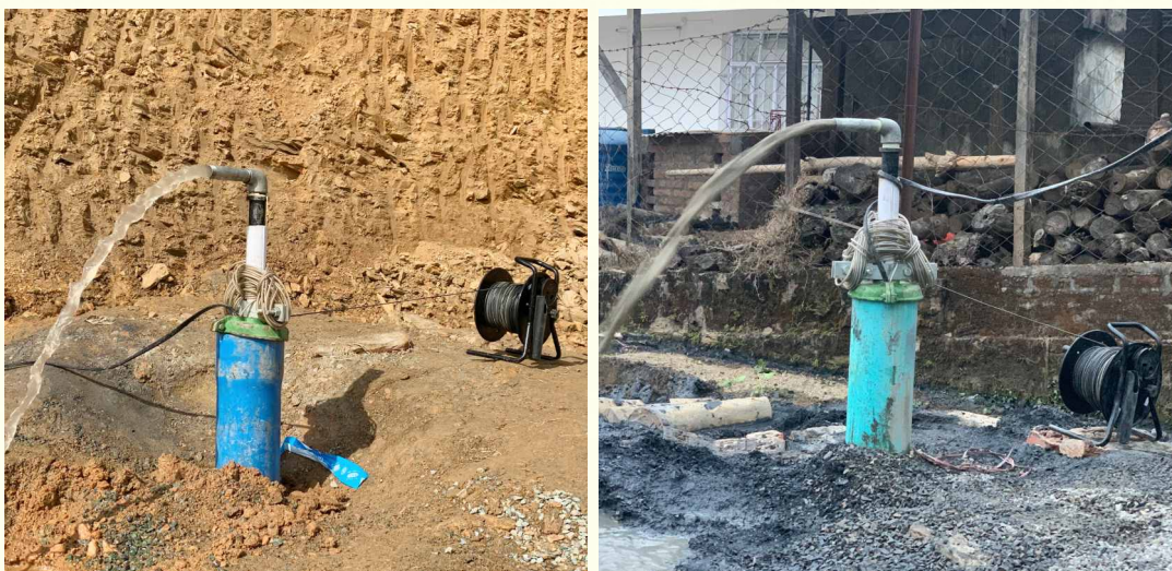
Pump test of a completed well in progress
