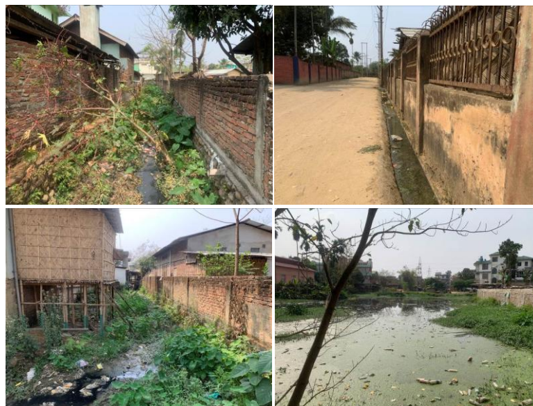
Pics: Clogged drains, absences of proper drainage system, encroachment of natural drainage and water bodies is contributing to inundation in urban areas.
